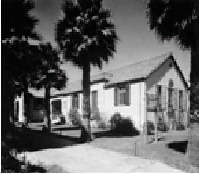
Exterior of Jefferson Park Branch Library 1928.
