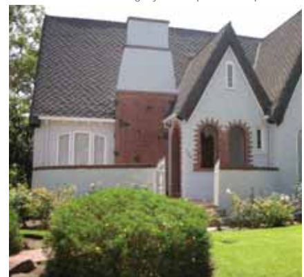
Not all homes will have porches. The garden wall and raised patio are appropriate for this English Revival Cottage. Garden walls may also be found on Spanish Colonial houses.
