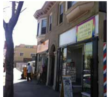
Many upper-floors on Jefferson Boulevard commercial structures are accented by dual bay windows.
