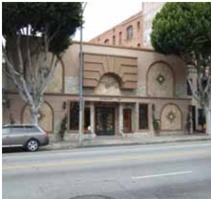
Pre-cast concrete, foam plant-ons and other similar materials are inappropriate on historic buildings.
