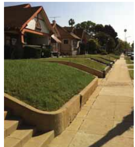
Historic retaining walls- often comprised of concrete or Arroyo Stone, are an important part of the neighborhood setting.
