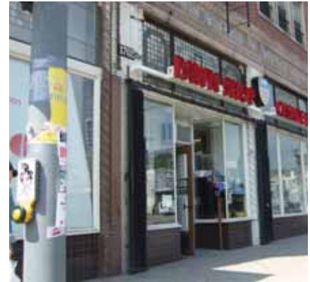
Individually cut channel letters, mounted to a canopy, allow for the transom window to remain open.
