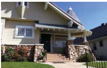
Porches are a significant part of the Jefferson Park neighborhood. This porch uses battered stone piers and a fanciful turet and is accented by exposed rafters-
