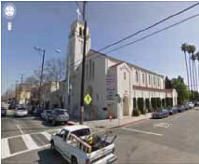
Westminister Presbyterian Church at the corner of Jefferson and 3rd Avenue.
