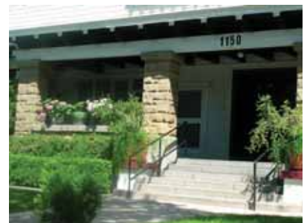
The sandstone porch columns are left to display their natural finish quality.
