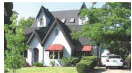
This second-story addition, with its noticable dormers, calls attention to itself, overwhelming the original cottage.
