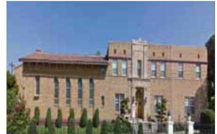
Sister Servants of Mary Convent located at 2131 W 27th Street, built in 1931.
