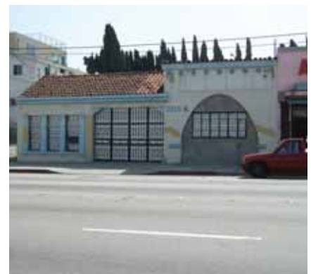
Concrete block is not a material that is original to this Spanish Colonial building.
