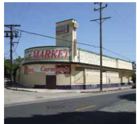
Doors and windows have been removed from this building (in favor of a rear-facing parking lot), to the detriment of the street.
