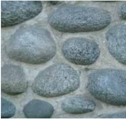
Wood clapboard, concrete and stone are all historically appropriate materials. When replaced, care should be taken to replicate texture, arrangement and dimension.
