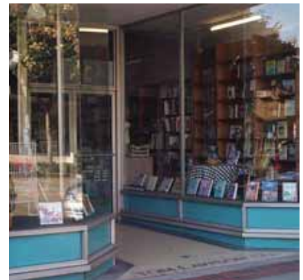
Bulkheads allow for storefront displays as well as the placement of durable and decorative materials along the storefront.
