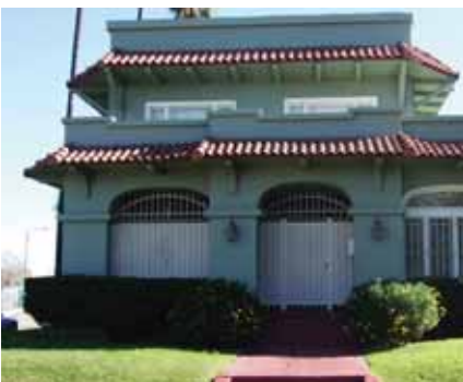
Enclosing a front porch disrupts the porch's intended purpose as an outdoor room.
