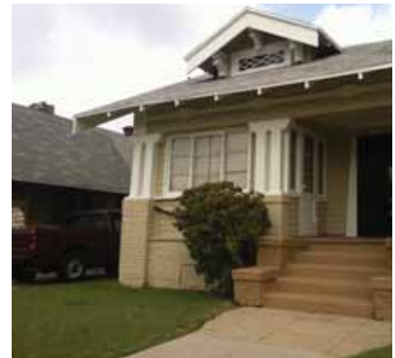
A portion of this porch has been enclosed in a manner that preserves the overall integrity of the porch components.
