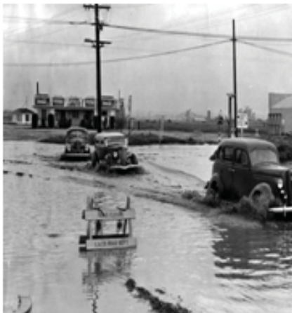
Flooded Jefferson Blvd. near Centinela 1941
