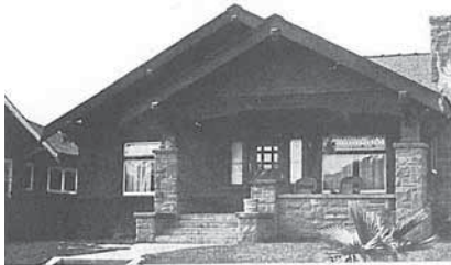
A SMALL CALIFORNIA BUNGALOW SHOWING THE USE OF RED PILLARS, PORCH FOUNDATION
