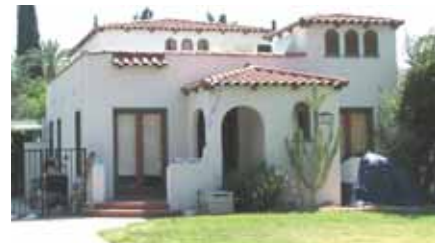
This second-story addition is set-back and preserving the look and scale of the original bungalow.
