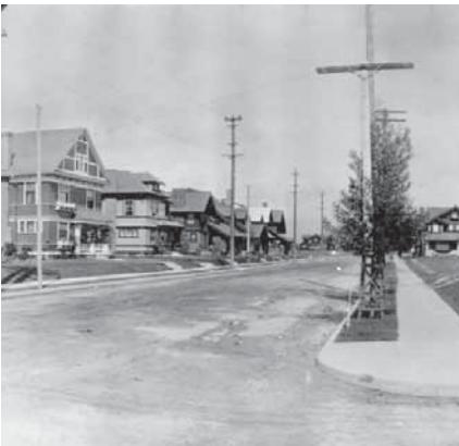
A collection of early Craftsman and Foursquare homes is shown in the Harvard Heights neighborhood (Western Ave. north of Venice Blvd.)
