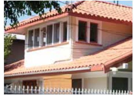
Clay tile is an inappropriate material for this Craftsman style home.
