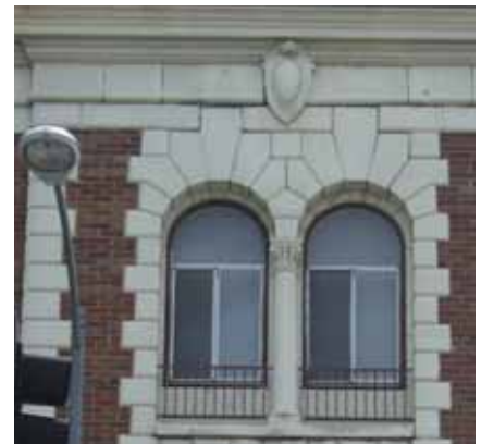
Pilasters, quoins and lintels are used on this building facade.
