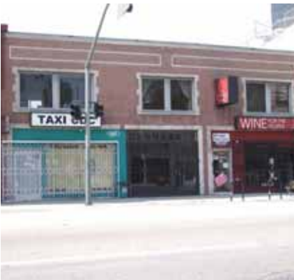
These storefront improvements are not appropriately sized to their bays.
