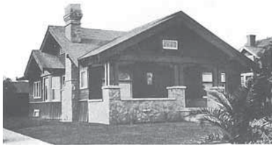
BUNGALOW BUILT FOR $1,900; INTERESTING SIMPLY WOOD CONSTRUCTION, WITH POCORATION, PORCH AND SOUTH WALLS OF WHITE LIMESTONE
