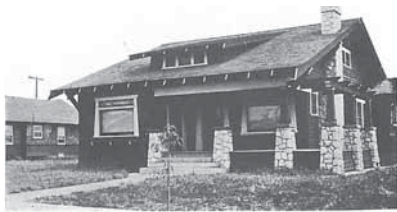
$2,500 CALIFORNIA COTTAGE WITH UNUSUAL WINDOW ARRANGEMENT IN THE ROOF AND WITH PICTURESQUE PORCH PILLARS AND CHIMNEY OF LIMESTONE.
