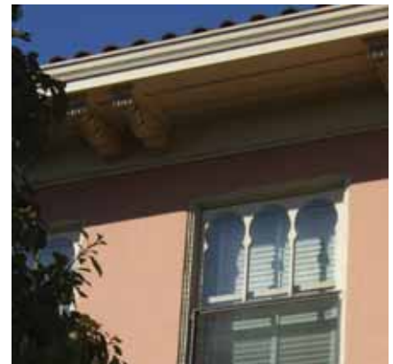
Smooth, hand-trowled stucco is an appropriate finish for this Italian Renaissance Revival home.
