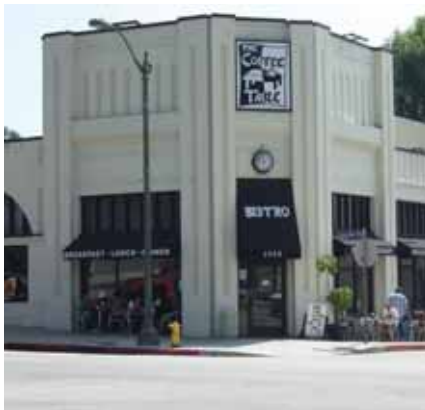
This plaster facade provides vertical ridges.
