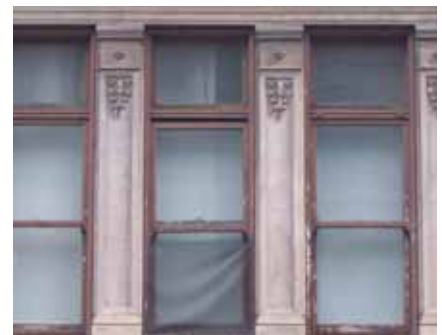
These windows should be repaired rather than replaced.
