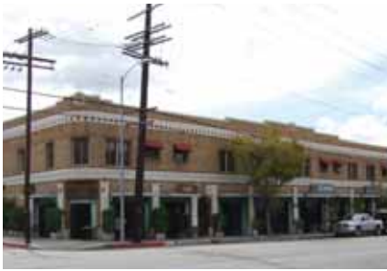
The upper-floor windows have not been filled-in and maintain a cohesive fenestration pattern.
