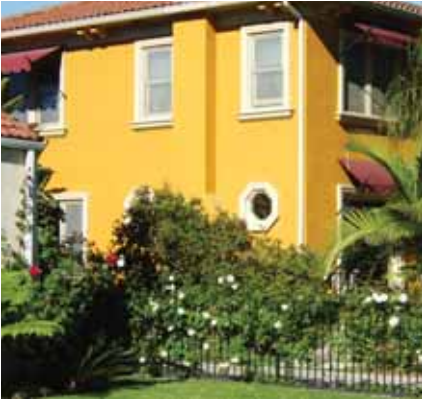
Foam plant-ons and pre-cast concrete are materials that would not have been originally used on this historic house.
